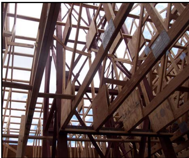
Figure 2: Roof trusses of 2x4 No.2 Southern Pine spaced at 2' OC. 1
