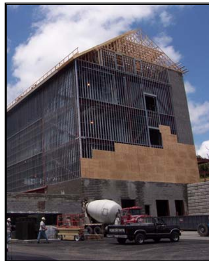
Figure 3: Light gauge steel framing with plywood sheathing 1
