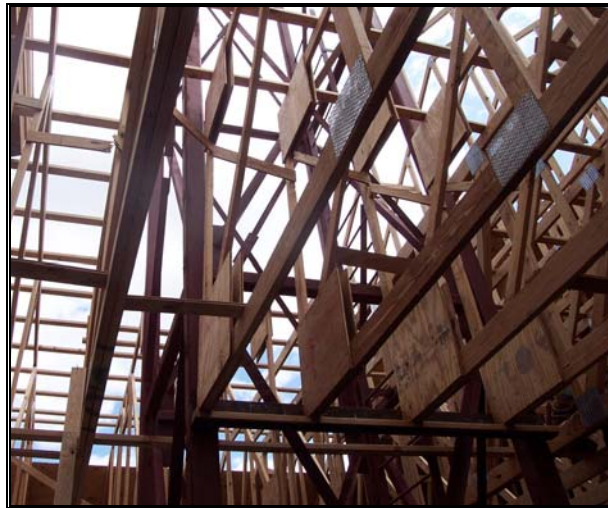
Figure 2.04: Roof trusses of 2x4 No.2 Southern Pine spaced at 2' OC. 1
