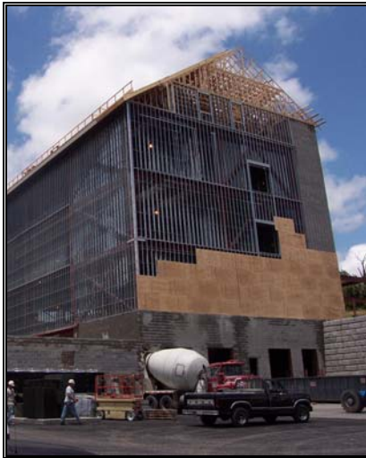
Figure 2.03: Light gauge steel framing with plywood sheathing 1
