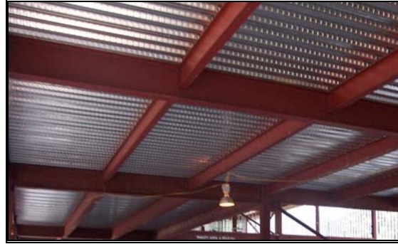
Figure 2.06: Composite slab as placed during construction 1
