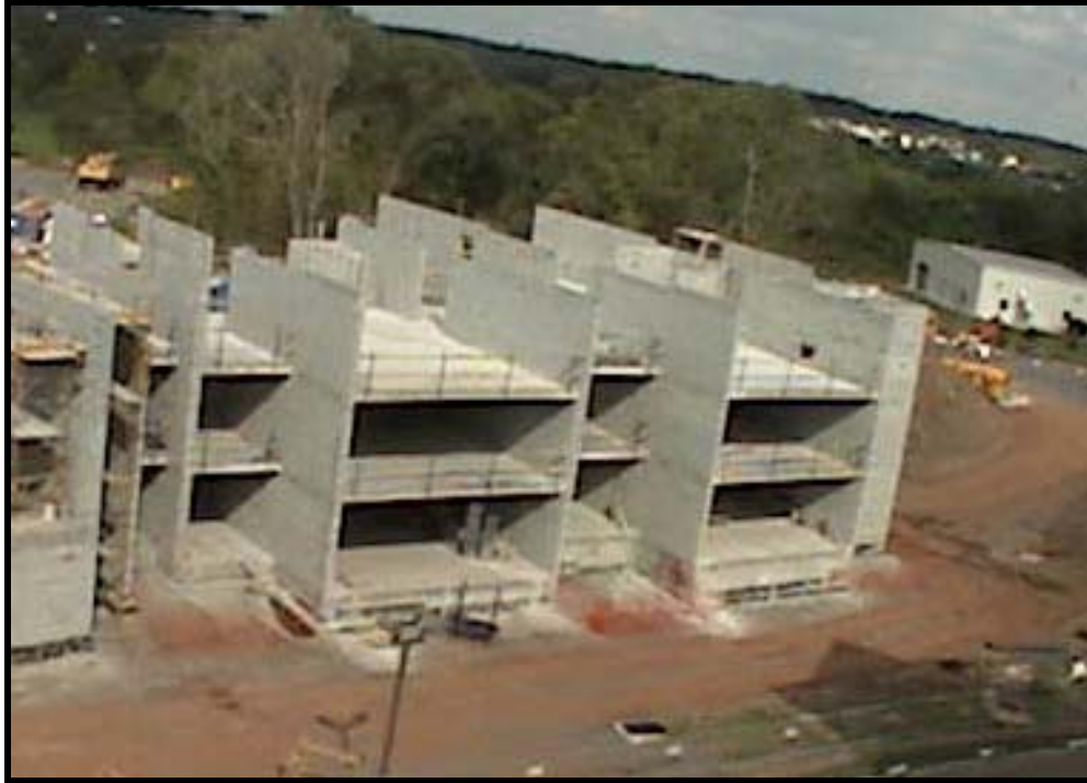
Residence Hall 2 During Precast Erection
