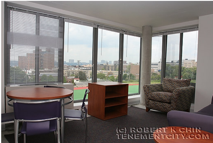
Figure 5: Photograph illustrating the concrete column obstructing the window (Photo courtesy of Robert Chin)
