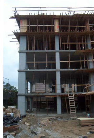
Figure 3: Concrete framing (photo courtesy GPI)
