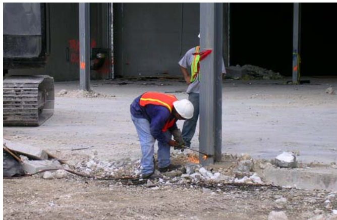
F8. Column Torching For Demolition
