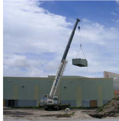
F1. RTU Removal for future re-installment
