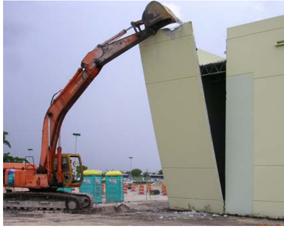
F3. First Panel Removed on West Wall.
