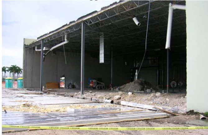
F6. West Wall on Ground before Saw Cutting
