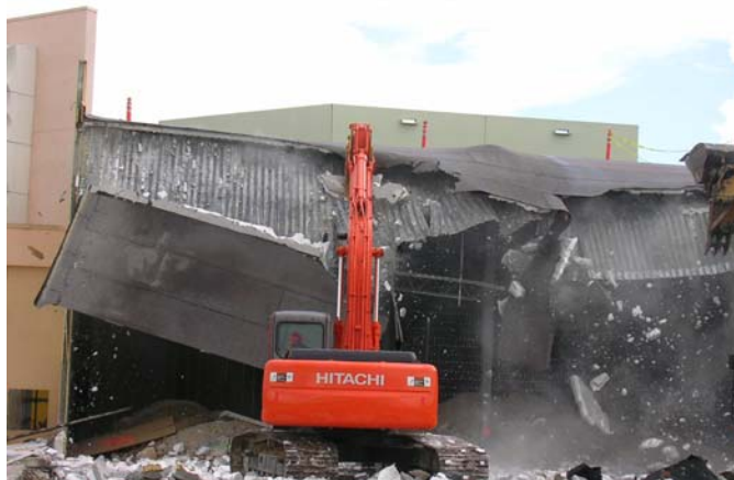
F7. Lightweight Concrete Roof Demolition
