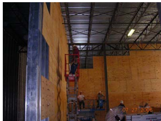
Fig. 4. "Hurricane Wall" Erection
