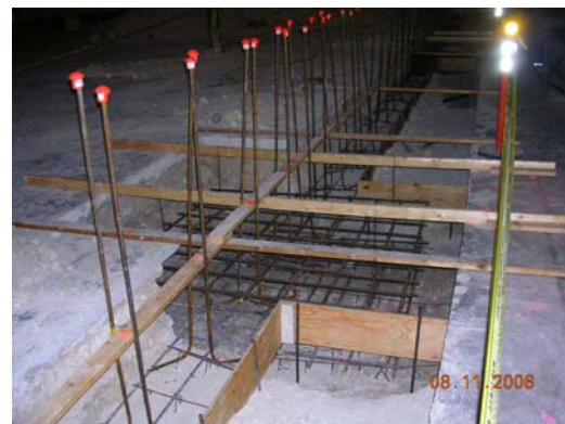
Fig. 7. Column Line "A" Footings
