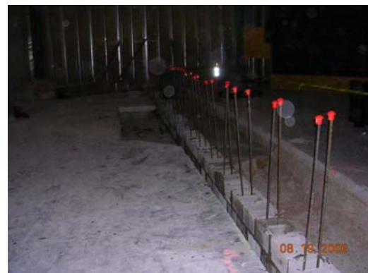
Fig. 8. Masonry Before Demolition
