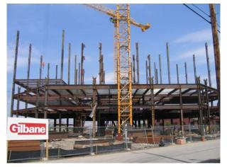
perimeter. The height of the tower cranes were 340 ft & 380 ft respectively. They have a concrete foundation with eight precast piles under each. The pieces of the cranes, known as "towers", were each approximately 20' tall. To remain structurally safe, the max free standing towers are nine or 180'. Once the cranes were above the 180' height limit, they
