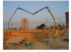
horizontal formwork for the concrete, while the steel toe plate around the perimeter will act as the vertical formwork. The concrete is to be poured in strips perpendicular to the steel girders. The cast in place concrete is placed by the pump method.
