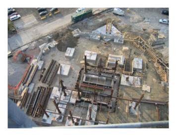
These pile caps are located on the column grid and each covers roughly 4-10 piles.
