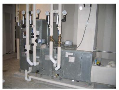
The mechanical design in the tower is based on two air handling units located on each floor. The units are constant volume vertical air units (8500 cfm), each consisting of mixing box, chilled water cooling coil
