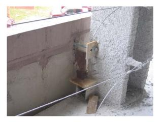
plates embedded in the concrete. The angles were attached to the structure columns and welded to embedded plates in the precast.
