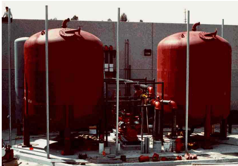
Cryogel Ice Ball system, exterior TES-Ice installation
