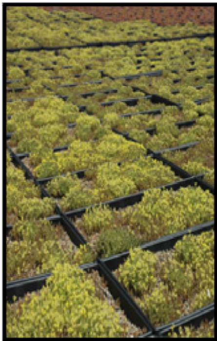
Figure 5 Modular GreenGrid System
