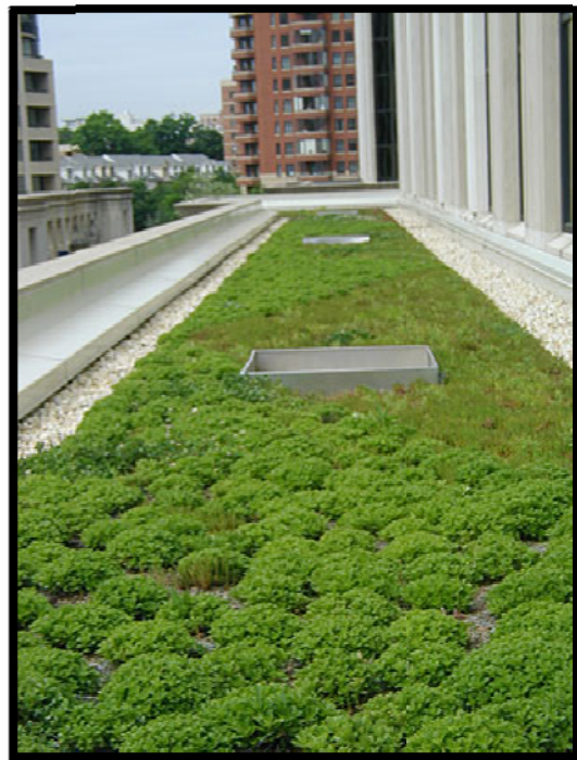
Figure 4 Typical Green Roof System
