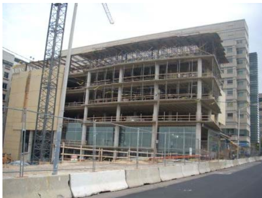
North face of the Outpatient Medical Center
