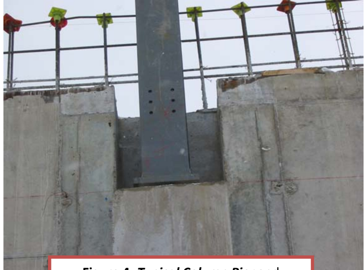
Figure 4: Typical Column Pier and foundation layout
