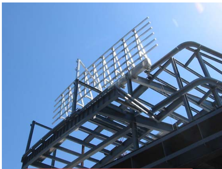
Figure 5: Penthouse Mechanical Screen with structural tube braces
