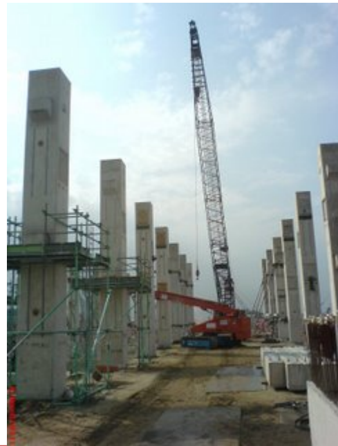
Figure 19: On-Site Picture of precast columns being erected
