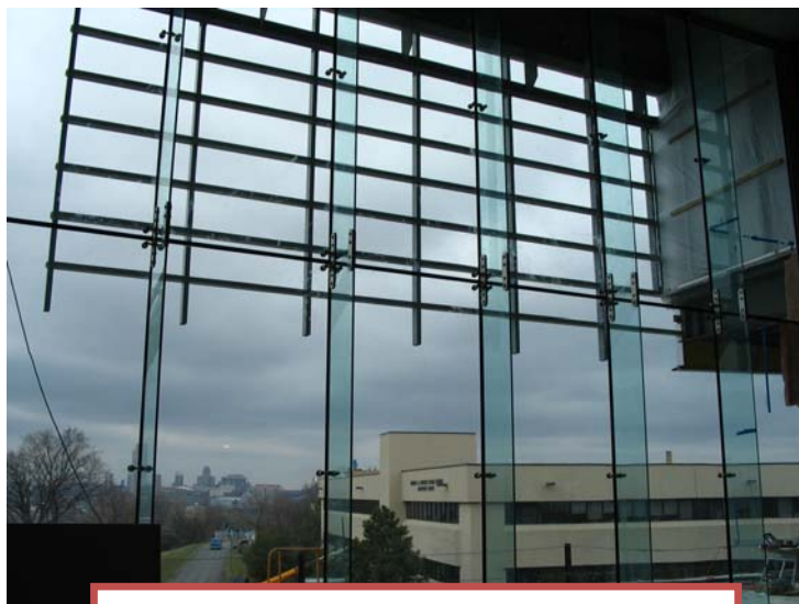
Figure 25: View from Behind Curtain Wall
