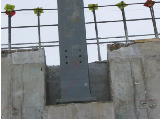
Picture 1: Typical Structural Column on Pier
