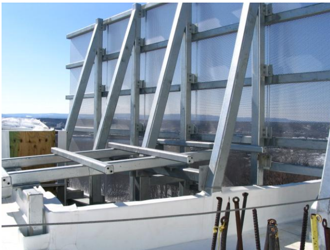
Picture 6: Penthouse Mechanical Screen
