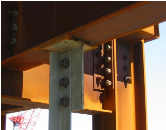
Picture 5: Typical Column-Girder Connection
