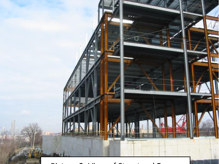
Picture 2: View of Structural Frame
