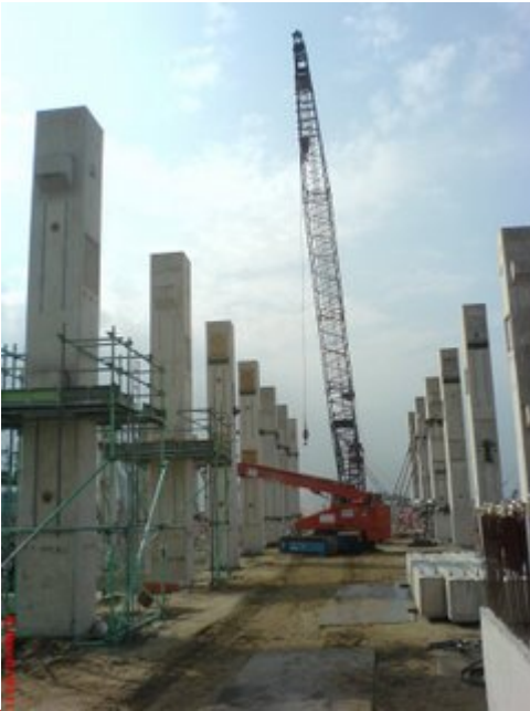
Figure 19: On-Site Picture of precast columns being erected
