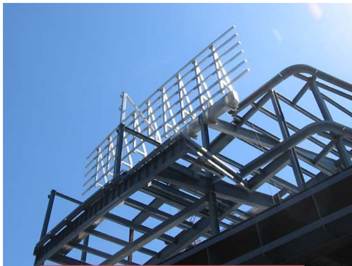
Figure 5: Penthouse Mechanical Screen with structural tube braces
