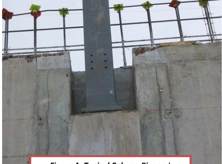
Figure 4: Typical Column Pier and foundation layout
