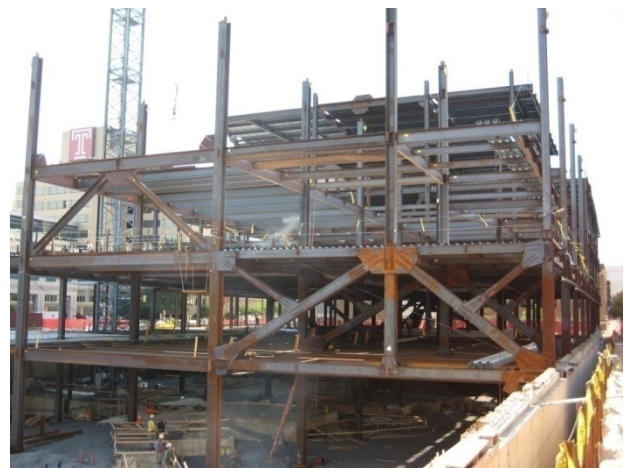
Figure 1: View of structural systems
