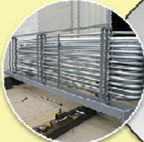
Prefabrication of piping which reduces installation time on the project site.
