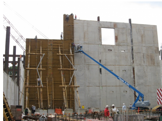
Figure 5.3: Pouring of concrete shear wall
