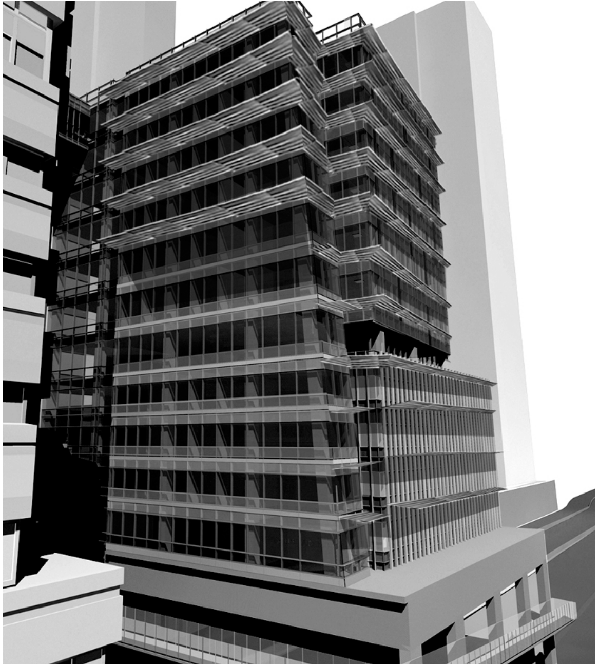
Figure 15. Southern exposure with solar shading system.
