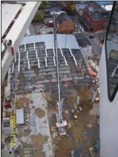
Photo from tower crane of crane erecting convention center steel.
