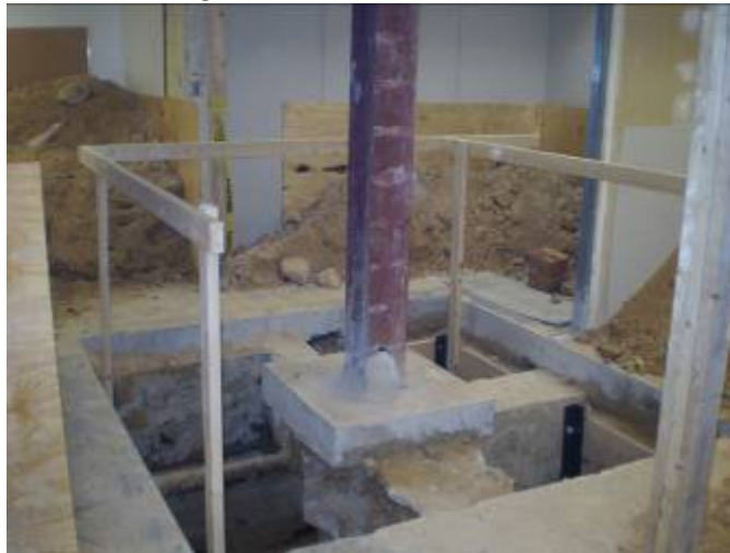
Figure 3: Excavation for Footing. Temporary Soil Storage with Wall Protection
