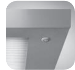
daylight / occupancy sensor
