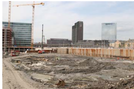
Figure14: Excavated Barcode site
