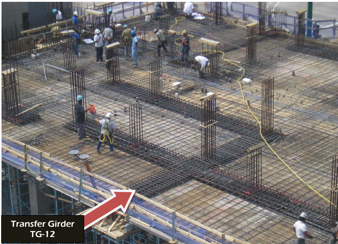
(FIGURE 7) Transfer Girder Reinforcing
