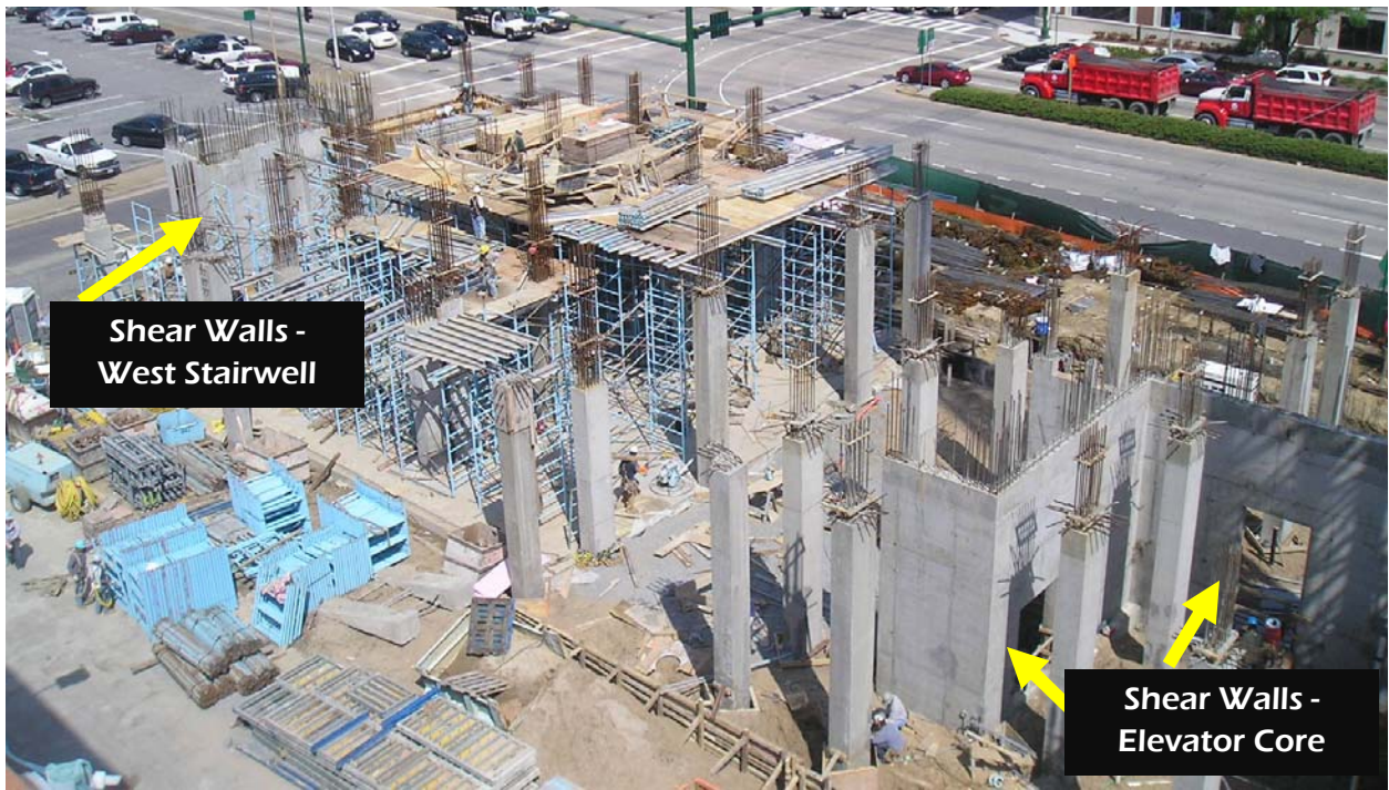
(FIGURE 14) Shear Walls & 1 st Floor Columns Under Construction
