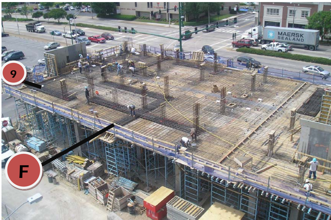
(FIGURE 8) West End 2 nd Floor Reinforcing Prior to Concrete Placement
