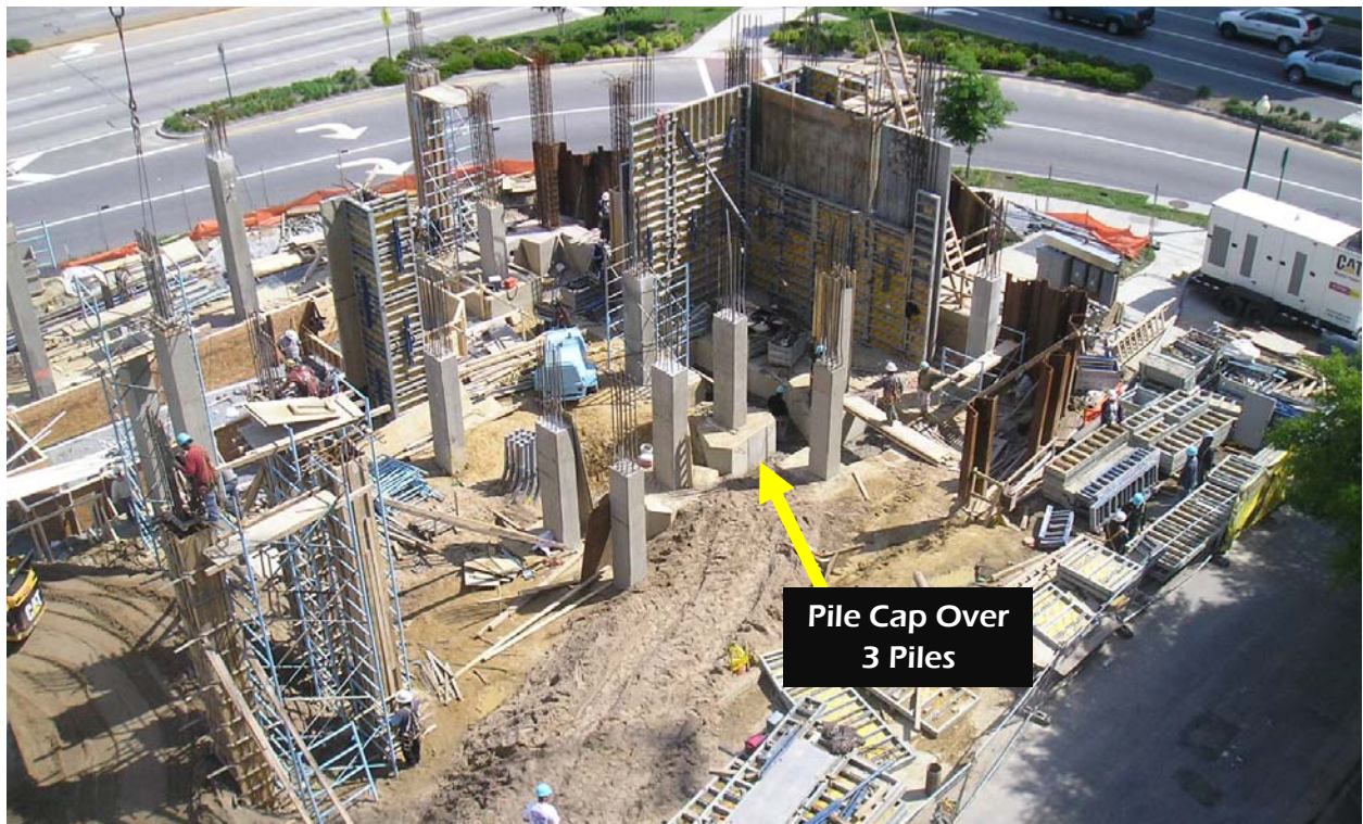
(FIGURE 3) Foundations & 1 st Floor Columns Under Construction
