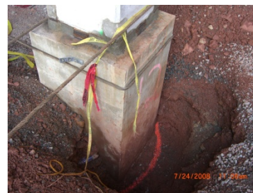
Figure 1 - - Temporary support for the sinking column E-12
