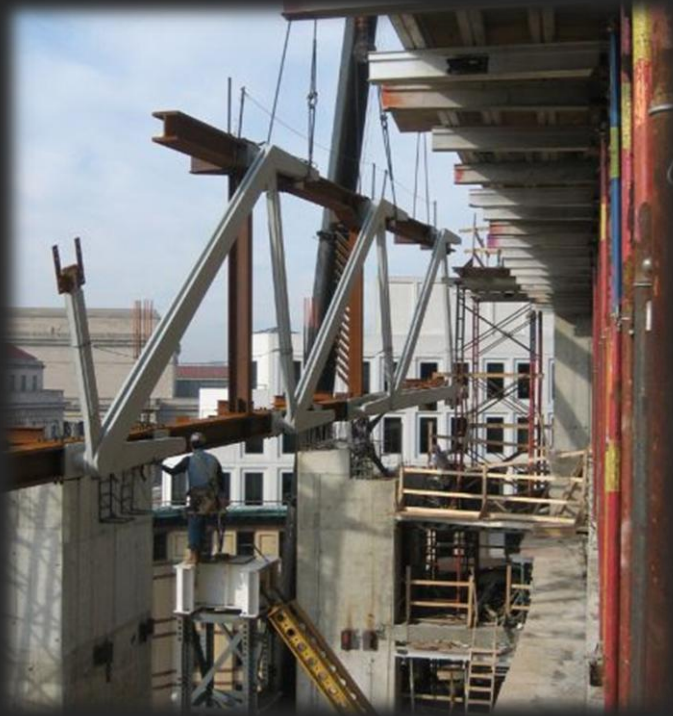
The Newseum "Megatruss"
