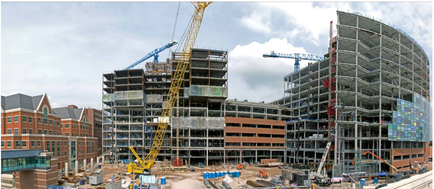
Figure 10: Typical Site Congestion
