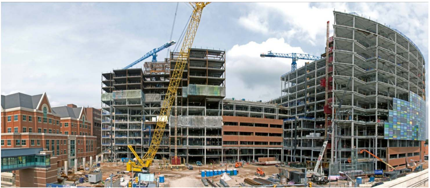
Figure 2: Typical Site Congestion
