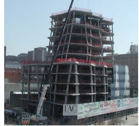
Figure 4: Photo taken during construction of superstructure
