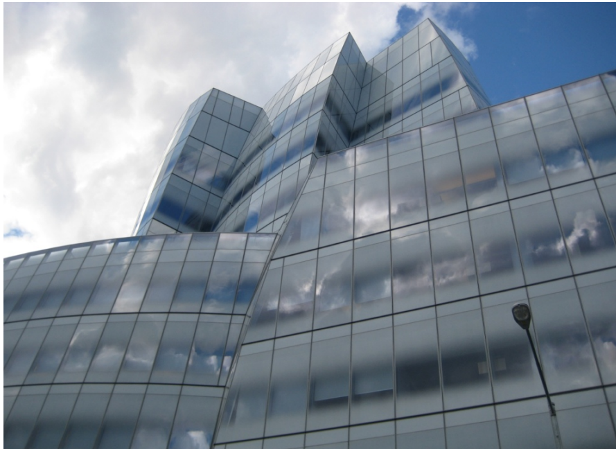
Figure C-2: Close-Up of building's curtain wall system
