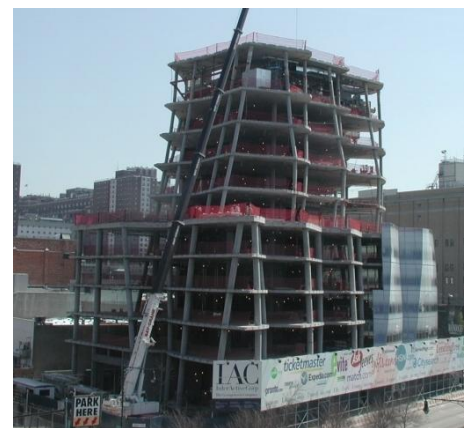
Figure 3: Flat plate system during construction of the IAC Headquarters
