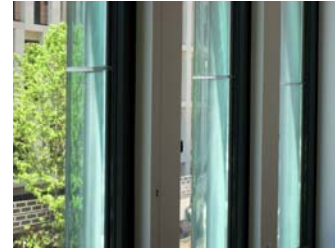
Figure 3 – Interior View of 10"×10" Columns within Glass Mullions
