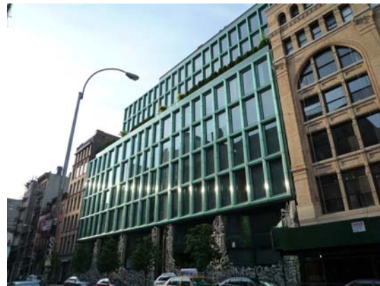
Figure 12 – 40 Bond and Neighboring Buildings
