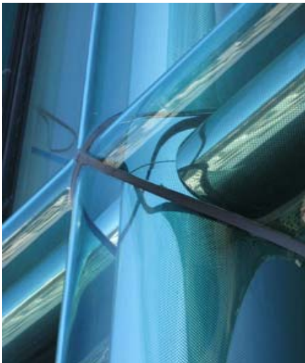
Figure 14 – Typical Mullion Intersection
