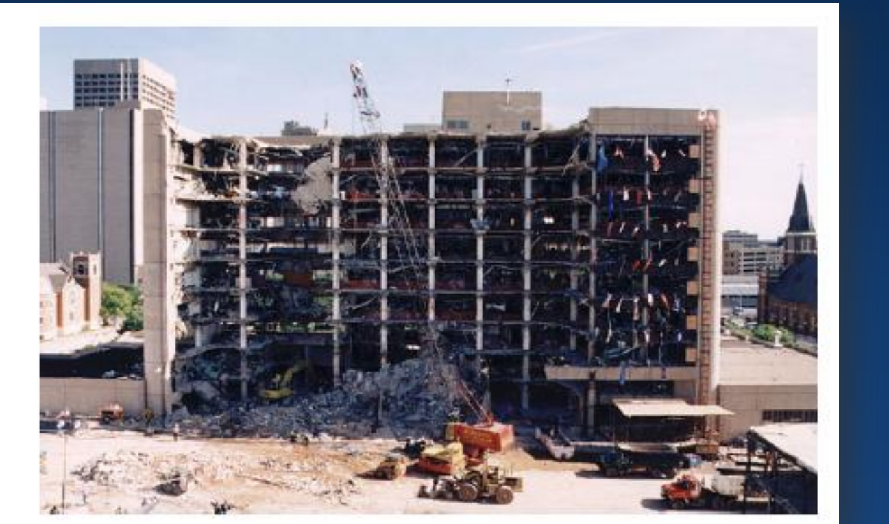
*MURRAH FEDERAL BUILDING – PORTION OF BUILDING COLLAPSED AFTER BEING BOMBED ON APRIL 19 TH , 1995
