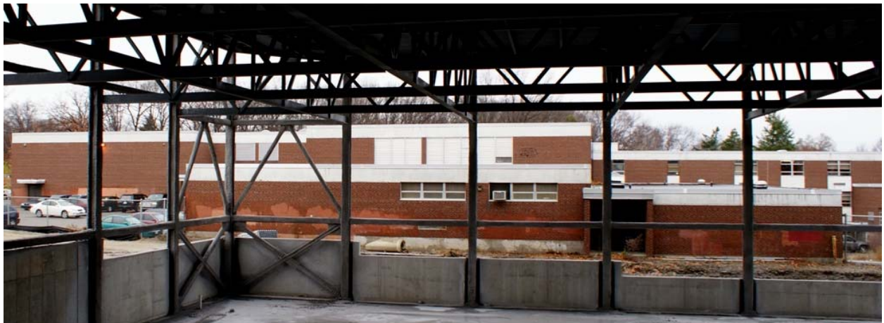
Figure 2A Gymnasium built in close proximity to existing building.
