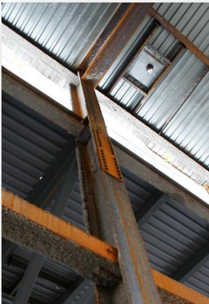
Column Splice at Gym/Auditorium
