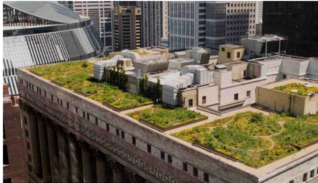
Figure 4 - Green Roof http://www.inhabitat.com/images/greenroofs1.jpg
