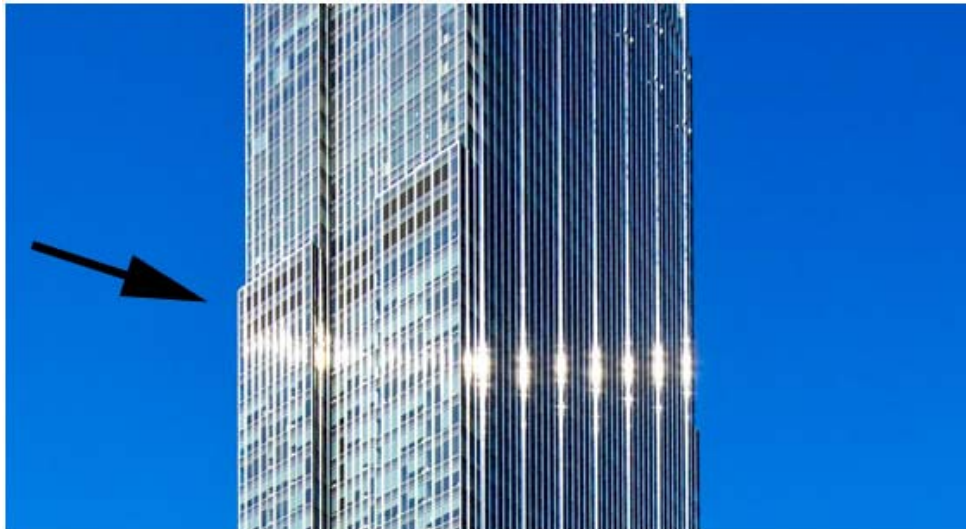
Figure 3: Noticeable change in façade at truss levels.
