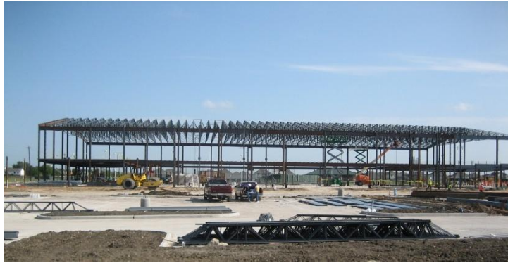
Figure 4-2.6 - Construction photo of roof trusses at recreation center
