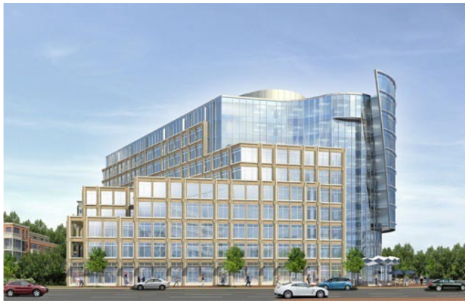
Figure 5: South East Face
