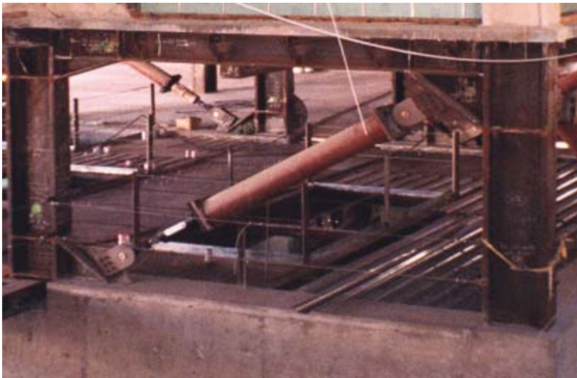
Figure 7: Diagonal Brace FVD Configuration
