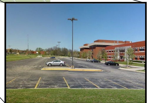
Figure 6: Camera View of the Existing Parking Lot and Adjacent Buildings
