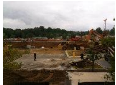
Figure 2: Parking Lot Demolition, July 13, 2010
