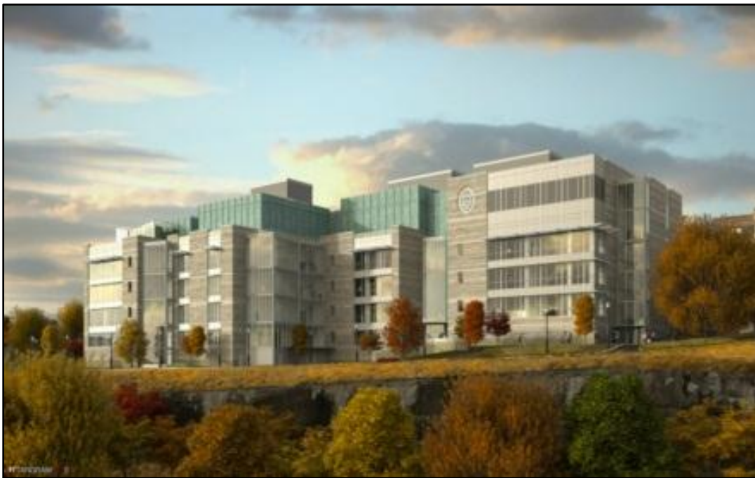
Fig. 29: South Façade View from Expressway
