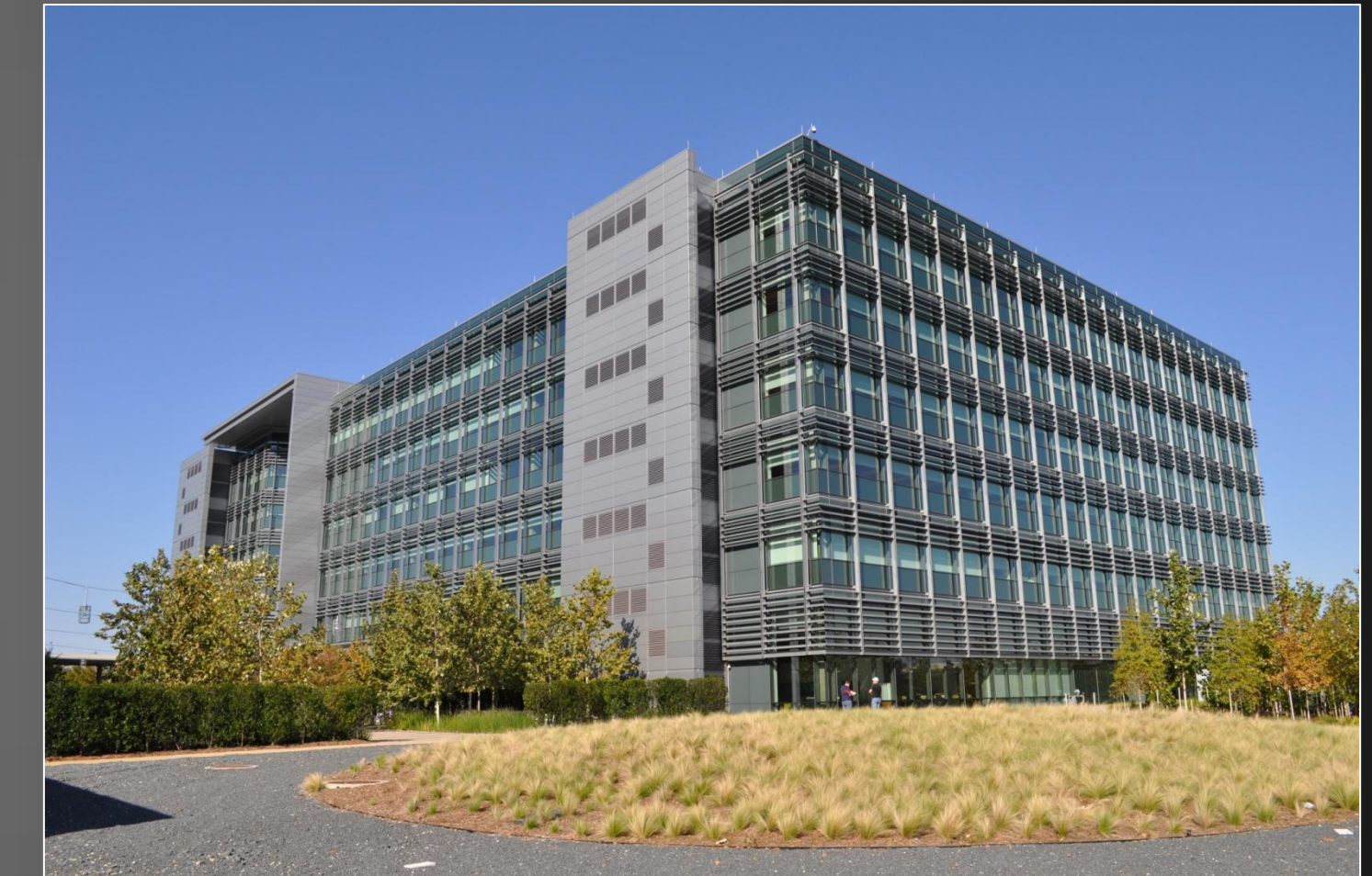
Exterior View of Southeast Corner
