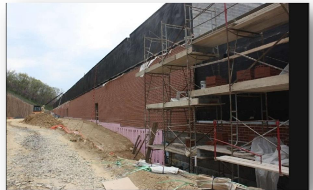
Fig. 4 Face brick facade construction
