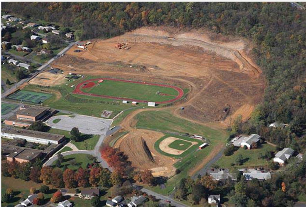
Fig. 7 Aerial View of site 10-26-08
