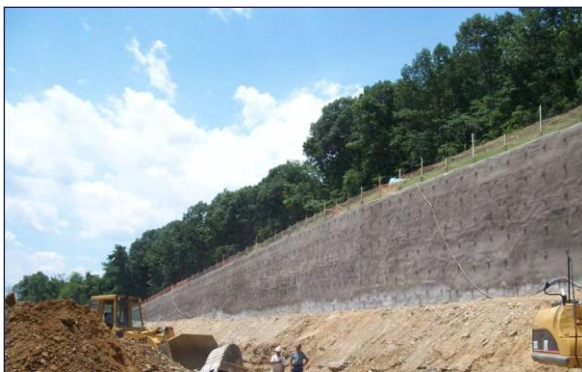
Retaining wall Pre-Finish
