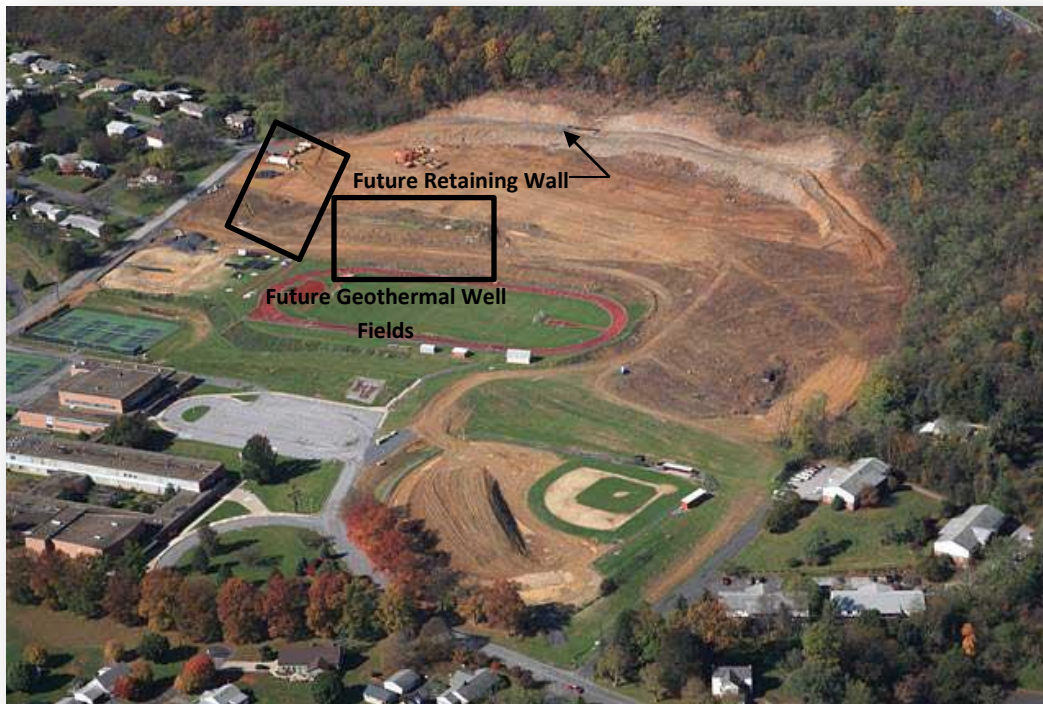
Excavation of site
