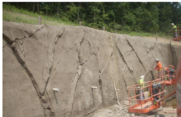
Retaining wall Post Finish
