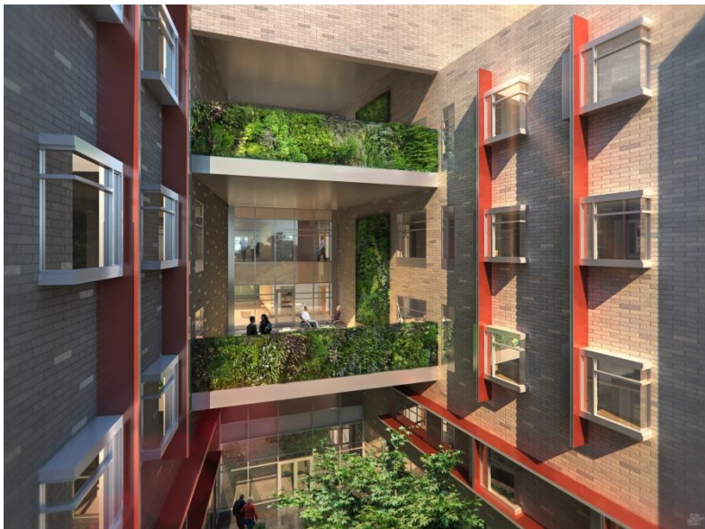
Figure 2: Exterior view of stacked garden terraces, green wall, and the building's vertical and horizontal shading panels. Rendering courtesy of Cannon Design.
