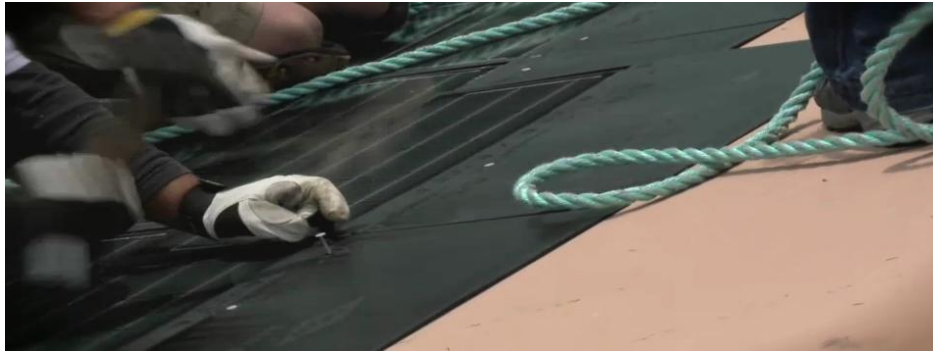
Figure 14: Solar Shingle installation using regular roofing nails (image property of DOW Chemical Company)
