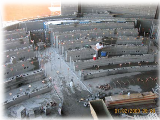
Figure 2: Installation of lecture hall structure
