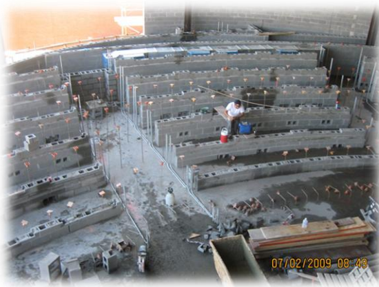
Figure 2: Installation of lecture hall structure
