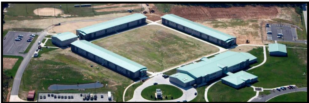
Figure 2: RTI Campus Courtesy of Barton Malow
