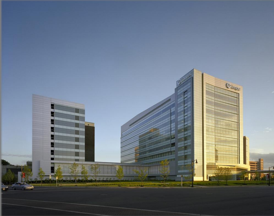
Roberts Pavilion Camden, NJ
